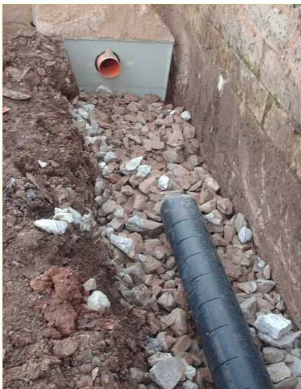
Fig. 4 – Posa in opera trincea drenante
