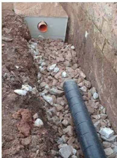
Fig. 6 – Posa in opera trincea drenante
