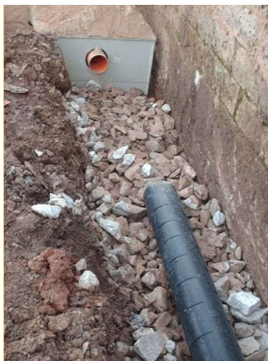
Fig. 6 – Posa in opera trincea drenante
