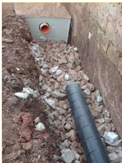
Fig. 6 – Posa in opera trincea drenante
