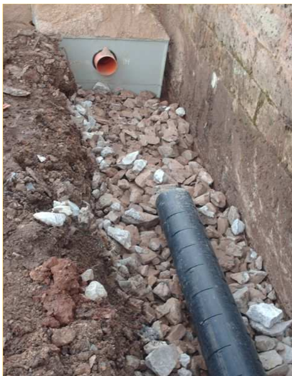
Fig. 4 – Posa in opera trincea drenante
