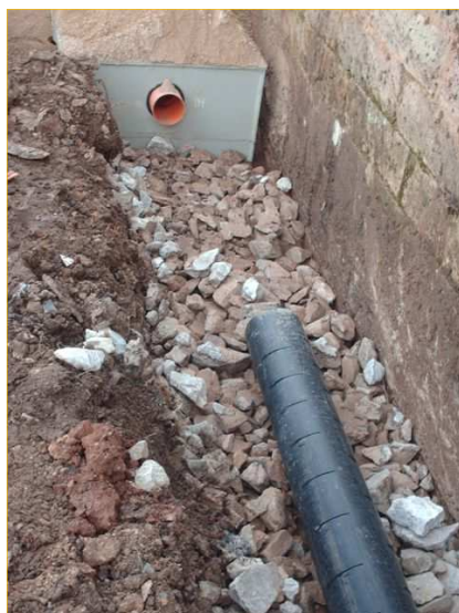
Fig. 6 – Posa in opera trincea drenante
