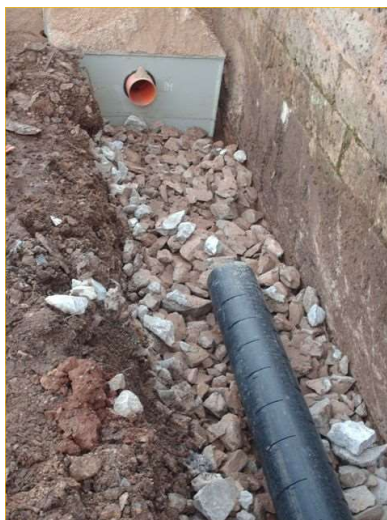
Fig. 6 – Posa in opera trincea drenante
